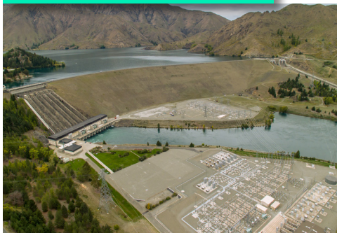
Benmore hydro station
