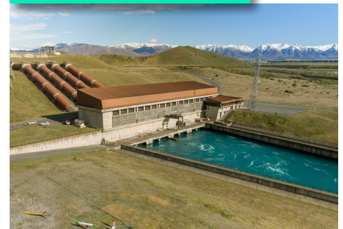
Ōhau B hydro station
