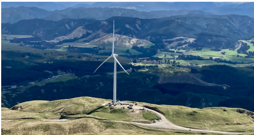
Our first turbine installed.
